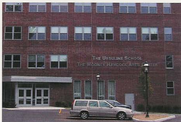
▶ Monte Brothers was recently commissioned to design and install a multi-purpose sound system as part of a 2-year, multimillion-dollar, 500-seat theater construction project at the Ursuline School in New Rochelle, NY.
